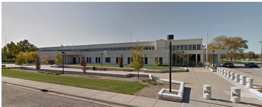
Police Building and Courts Building
