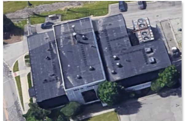
Dearborn central cooling plant
